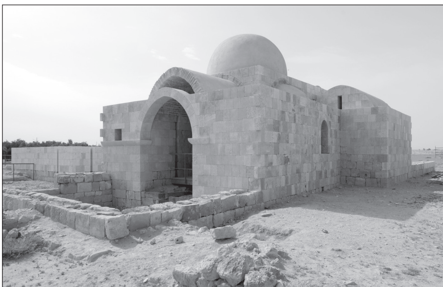
5. Qaṣr al-Ḥallābāt complex. The Umayyad bath-house of Hammam as-Sarraḥ, after restoration (photo by Dr. Arce).
